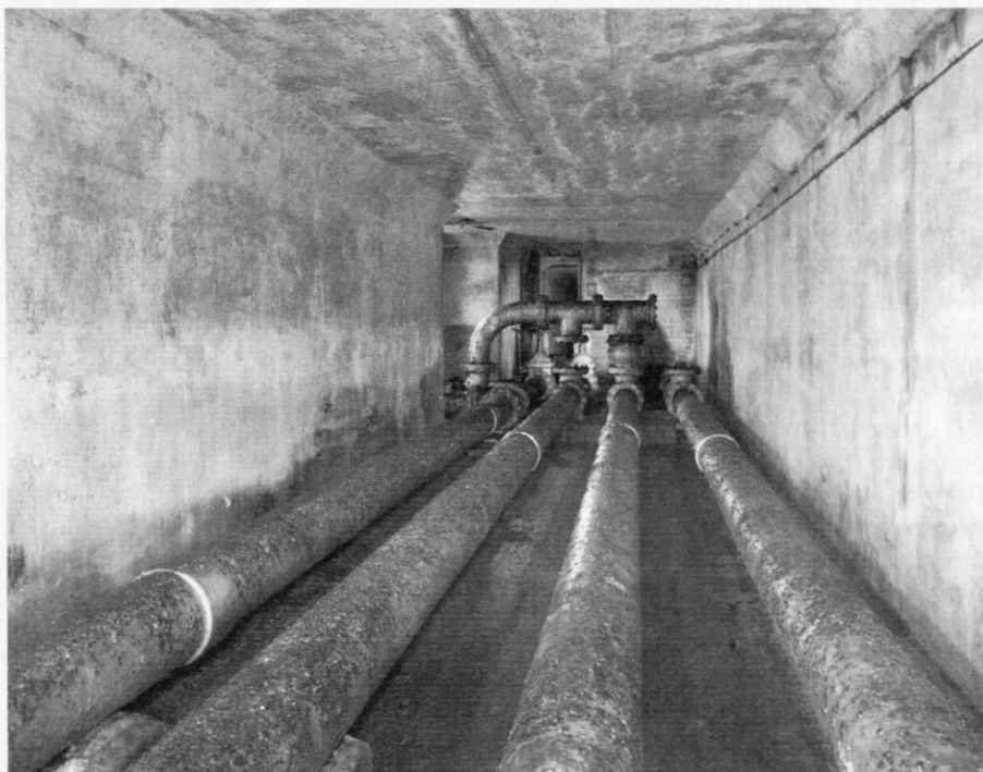
Milford Haven Underground Fuel Store - Photo Nick Catford
